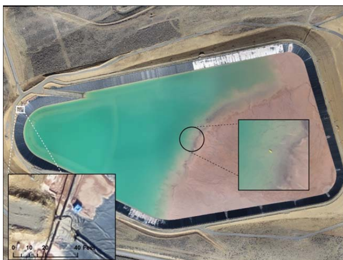
Figure 4. UAS imagery of tailings storage facility cell in northeastern Nevada. Inset on the right shows USV collecting data during the UAS flight. Inset on the left shows mine site infrastructure.
